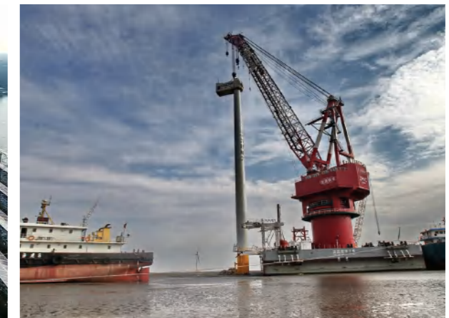
150MW offshore wind farm project in Indonesia
