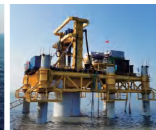
Hengtong seabed rock-socketed pile foundation drilling platform
