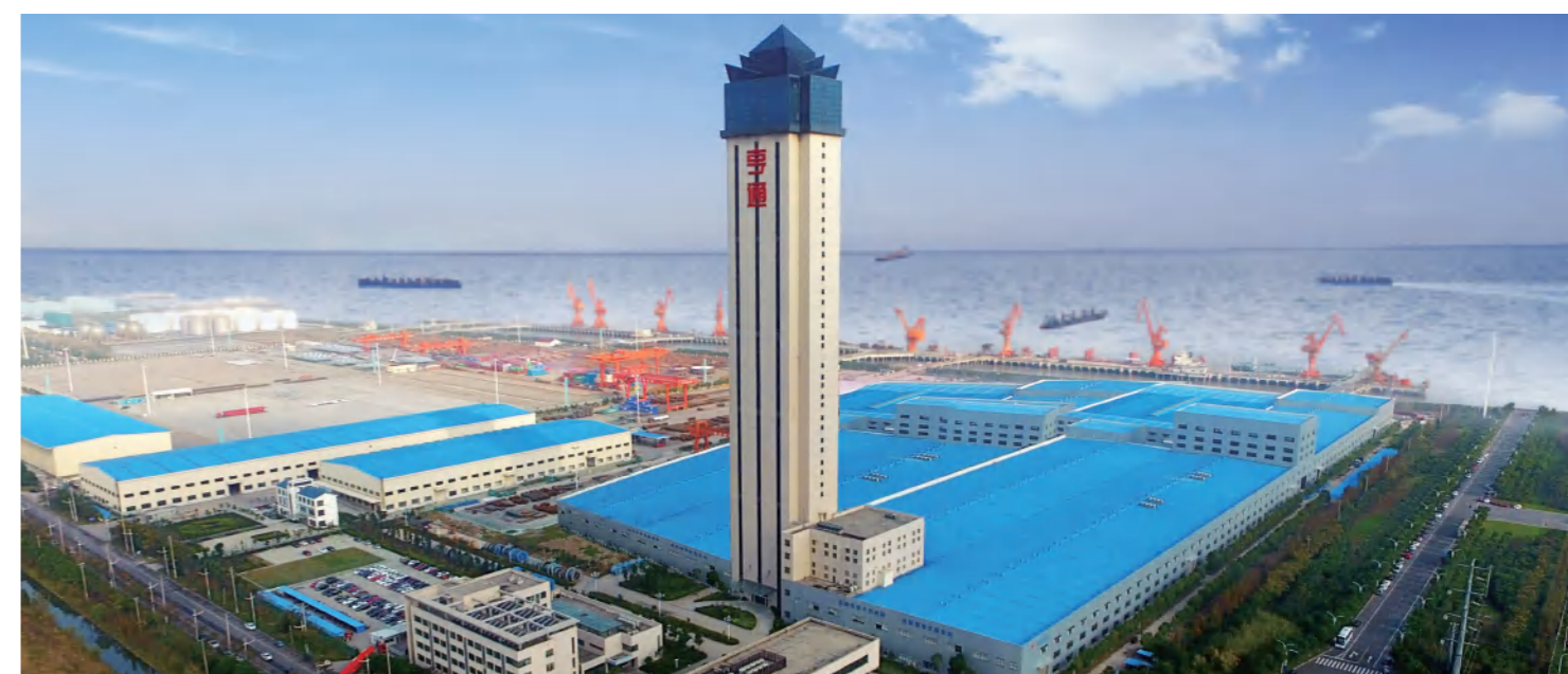
Hengton Submarine Power Cable Industry Park (Changshu City, Jiangsu Province, China)
