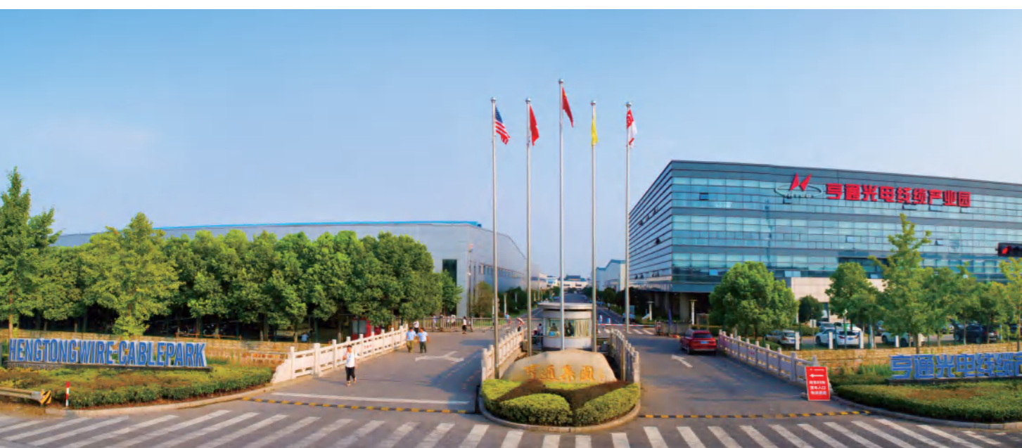
Hengton Wire&Cable Industry Park (Qidou Town, Suzhou City, Jiangsu Province, China)
